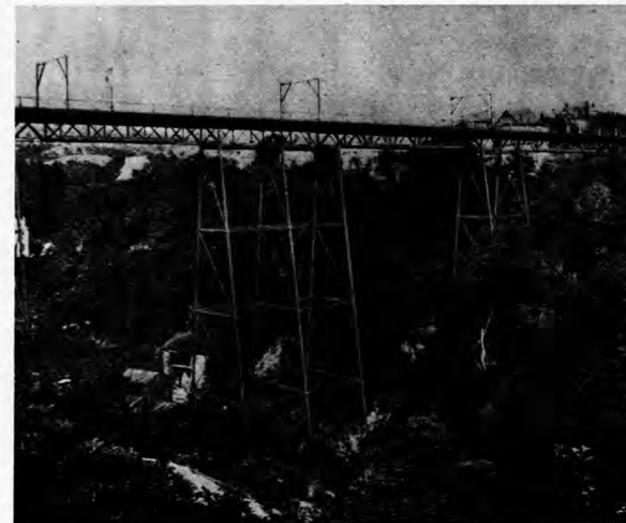
FIRST HIGH BRIDGE
