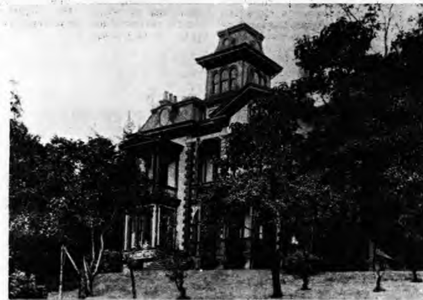
SUBURBAN GENERAL HOSPITAL - 1904
