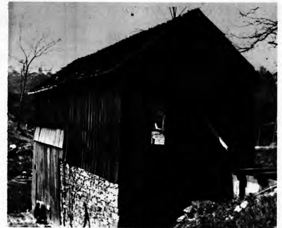
OLD SAW MILL on Spruce Run Creek at the foot of Home Avenue in Avalon and North Starr Avenue in Bellevue.
