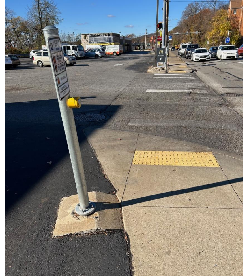
The southern leg of the Riverview Ave intersection. Tactile warnings and pedestrian push buttons are present, but crosswalk striping is in poor condition.
