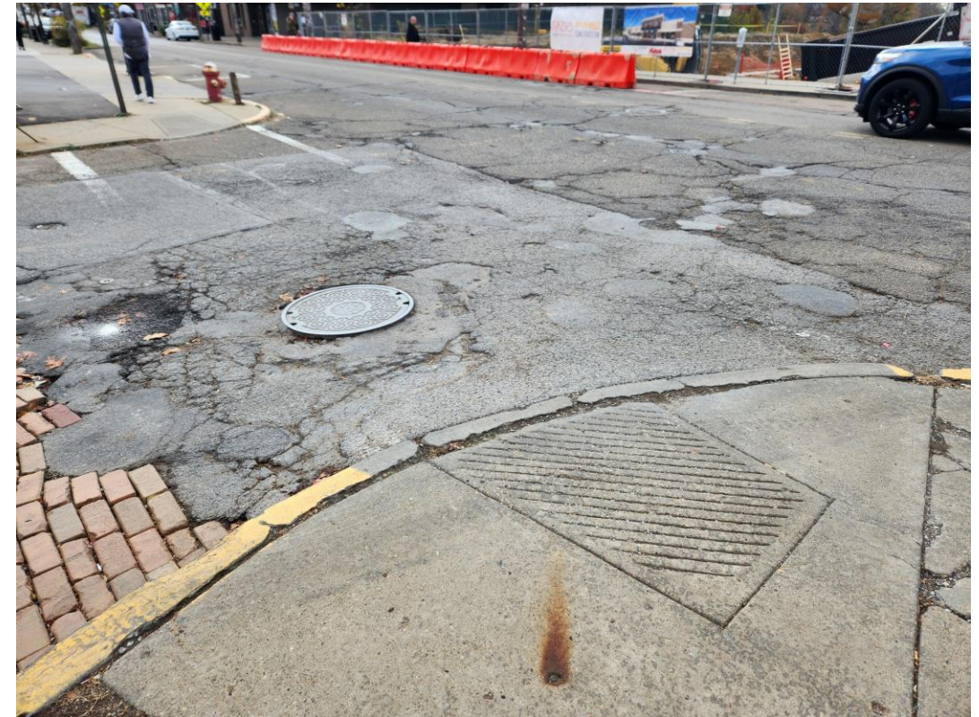
The intersection of Fremont Ave and Lincoln Ave, showing the poor condition of pavement and crosswalk striping to cross Fremont Ave.
