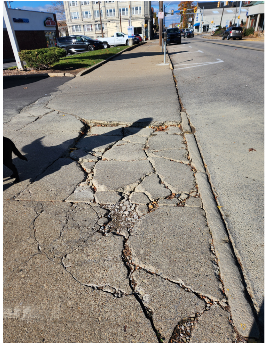
Image showing poor sidewalk pavement condition along the south side of Lincoln Avenue, near CVS. The surface condition of this sidewalk poses a barrier people using wheelchairs or other mobility devices, and may lead to them having to operate in the roadway.
